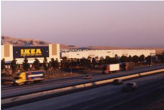
IKEA Distribution Center
